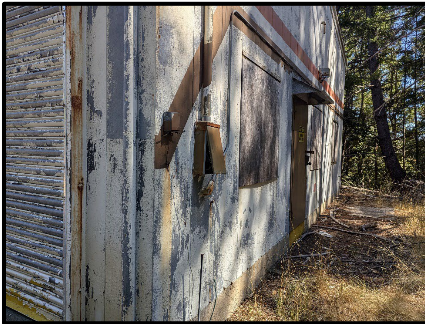
View of signage on southeast end of SS004, Building 217, former motor pool vehicle maintenance facility. No excavation of soil evident near building foundation. Building foundation intact and undisturbed.
