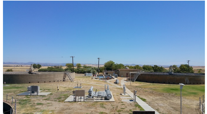
The Wastewater Treatment Plant at Beale AFB .
