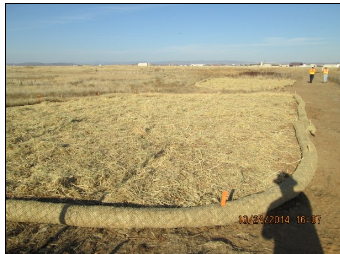
Straw wattles around graded and hydroseeded soil following soil pile removal at Site SD001.
