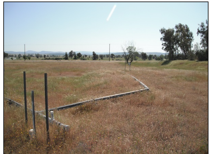
Soil vapor extraction infrastructure at Site FT029 prior to system decommissioning.
