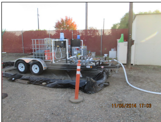
Site SS023 ISCO injection setup.
