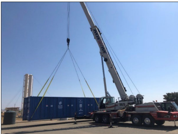
Crane setting the SAFF unit.
