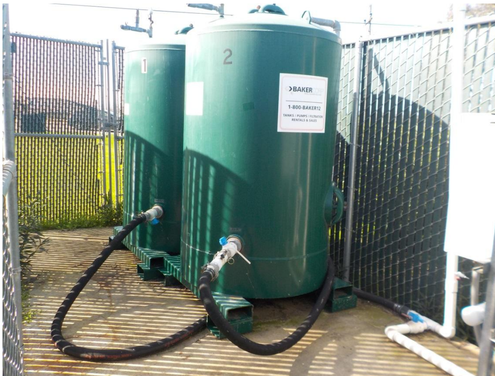
Photo 29 – TU002 Granular Activated Carbon Vessels
