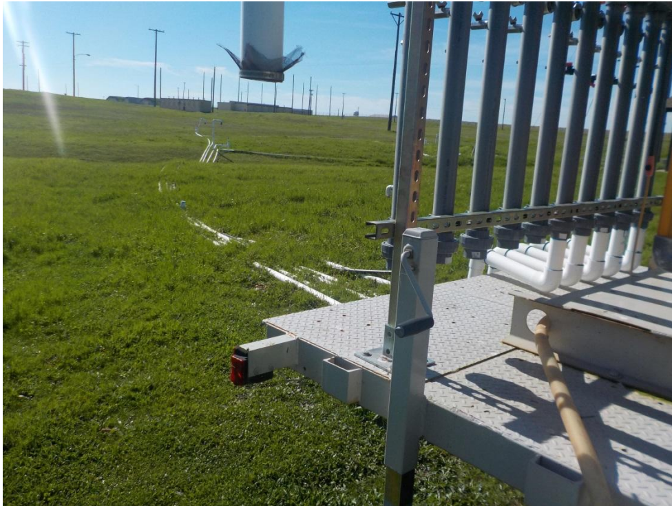
Photo 21 – SS035 SVE Conveyance Pipe to SVE Wells
