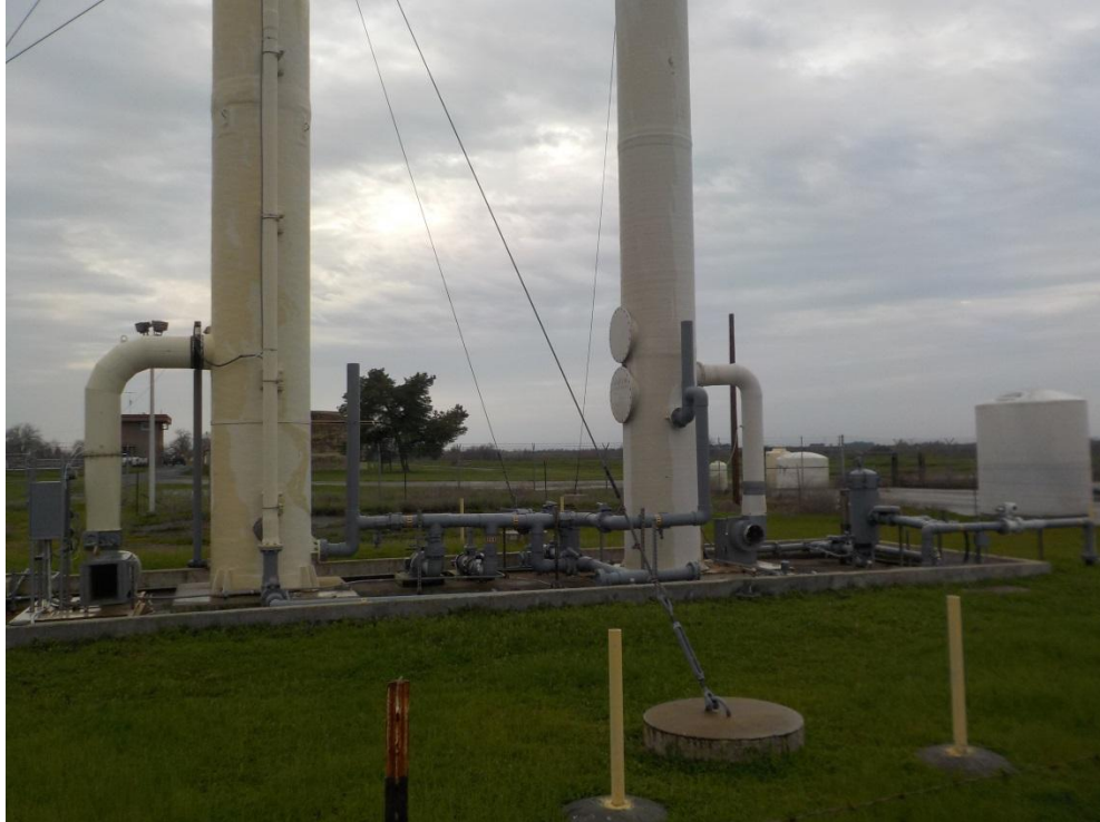
Photo 55 – CG041-013 Groundwater Treatment System (Air Strippers)
