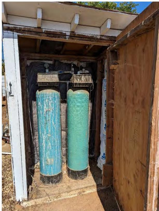
Photo C-31. Wellhead treatment system for off-Base residential well OBL005AW
