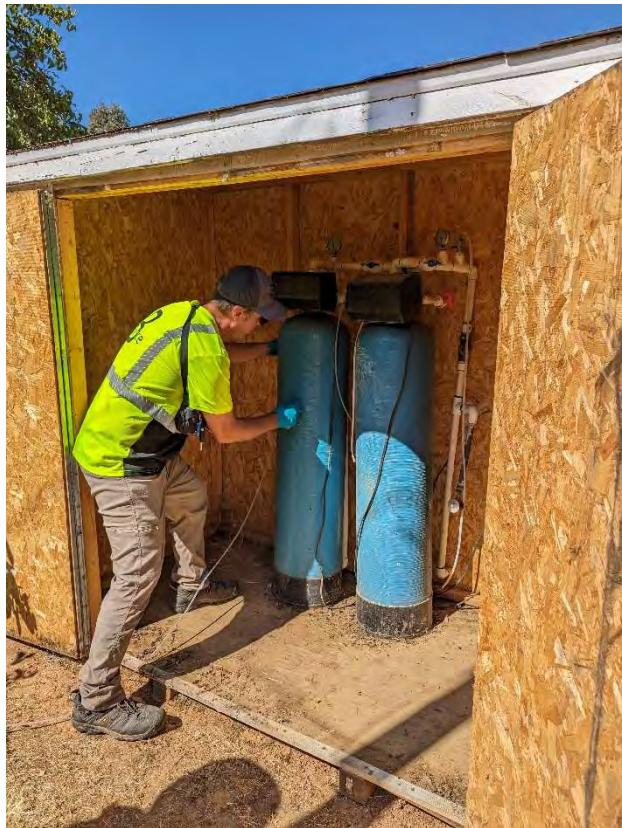
Photo C-30. Wellhead treatment system for off-Base residential well OBL004AW
