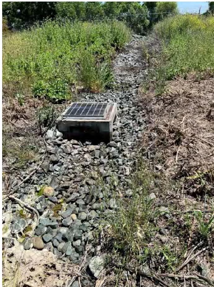
Photo C-24. CG044-013 – Hutchinson creek outfall for discharging GTS effluent
