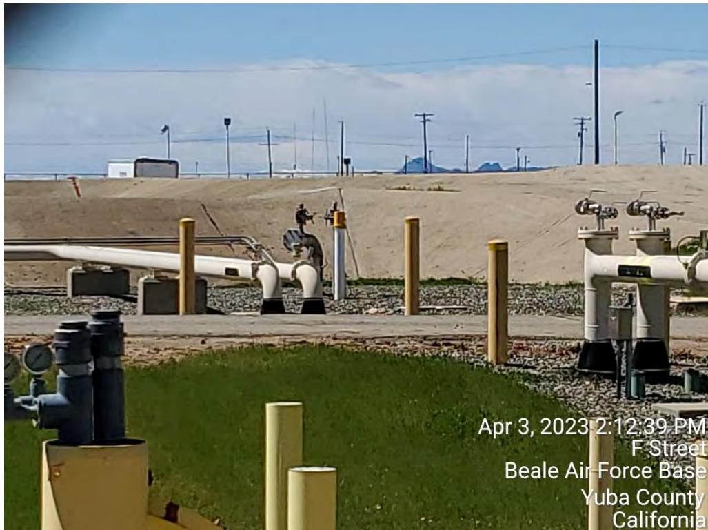
Photo C-7. CG041-018 – Well 18U007BMW (in the foreground to the left) with a passive skimmer for light nonaqueous-phase liquid recovery
