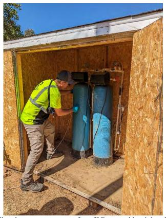
Photo C-30. Wellhead treatment system for off-Base residential well OBL004AW
