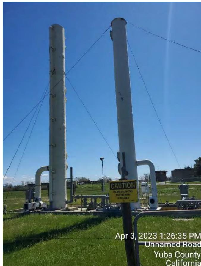
Photo C-16. CG044-013 – Groundwater treatment system with air strippers
