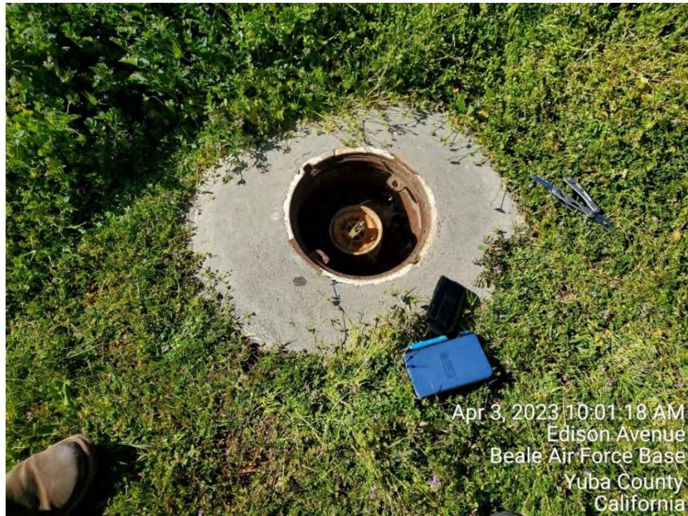
Photo C-29. CG044-032 (SD032) – Monitoring well intact; no signs of damage
