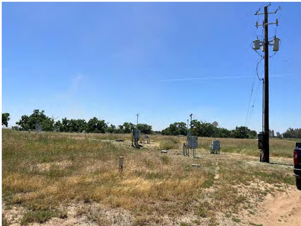
Photo C-20. CG044-013 – Groundwater wells and remnants of former SVE system
