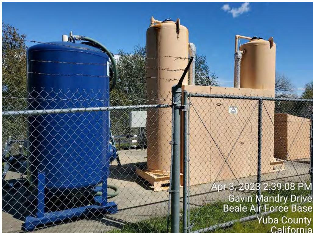
Photo C-4. CG041-017 – GTS with air stripping towers and the GAC vessel
