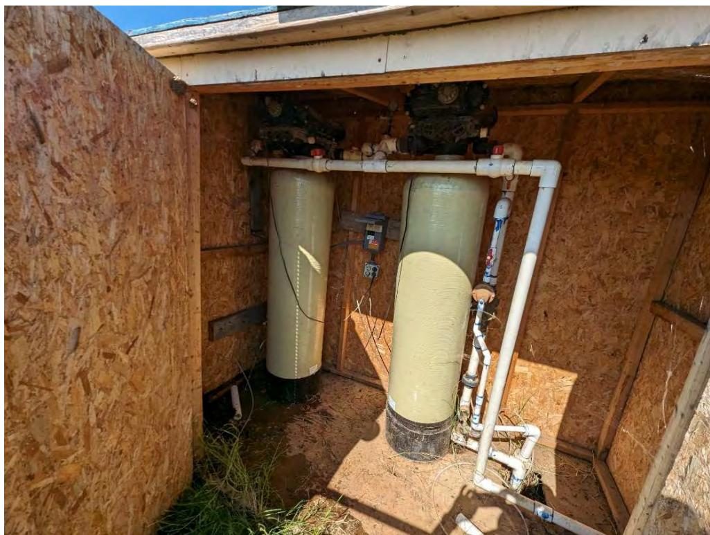
Photo C-32. Wellhead treatment system for off-Base residential well OBL008AW
