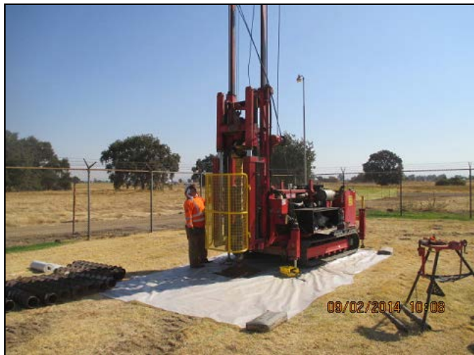
Hollow-stem auger drilling activities at Site PL582 during Summer 2015.
